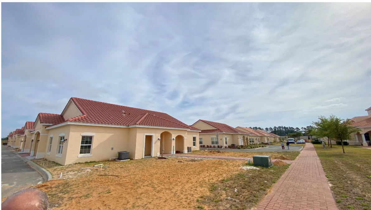
TYPICAL EXTERIOR VIEW OF SUBJECT RESIDENTIAL BUILDING
