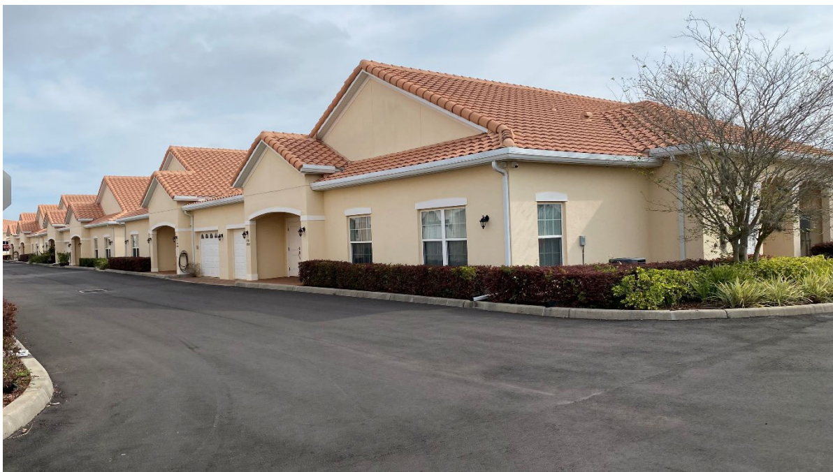
TYPICAL EXTERIOR VIEW OF SUBJECT RESIDENTIAL BUILDINGS
