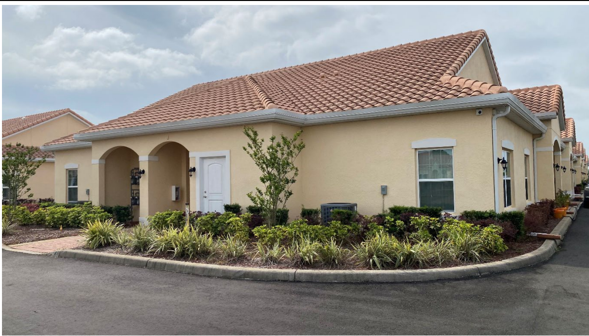
TYPICAL EXTERIOR VIEW OF SUBJECT RESIDENTIAL BUILDING
