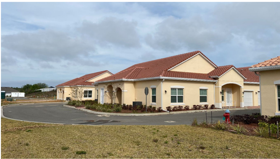
TYPICAL EXTERIOR VIEW OF SUBJECT RESIDENTIAL BUILDING
