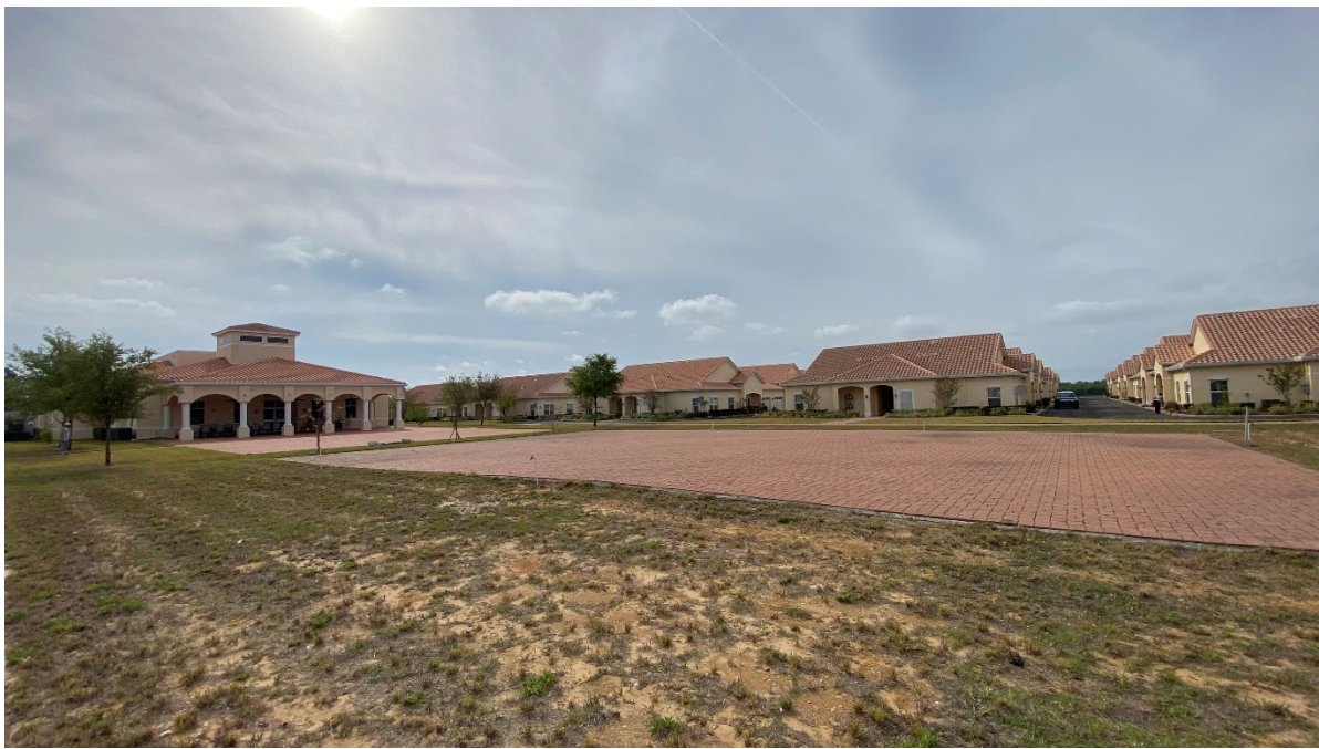
TYPICAL EXTERIOR VIEW OF SUBJECT RESIDENTIAL BUILDINGS
