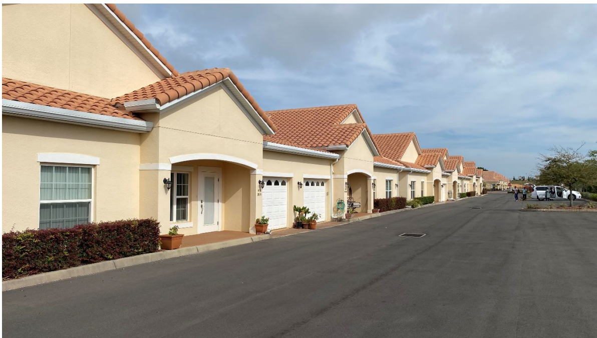
TYPICAL EXTERIOR VIEW OF SUBJECT RESIDENTIAL BUILDINGS
