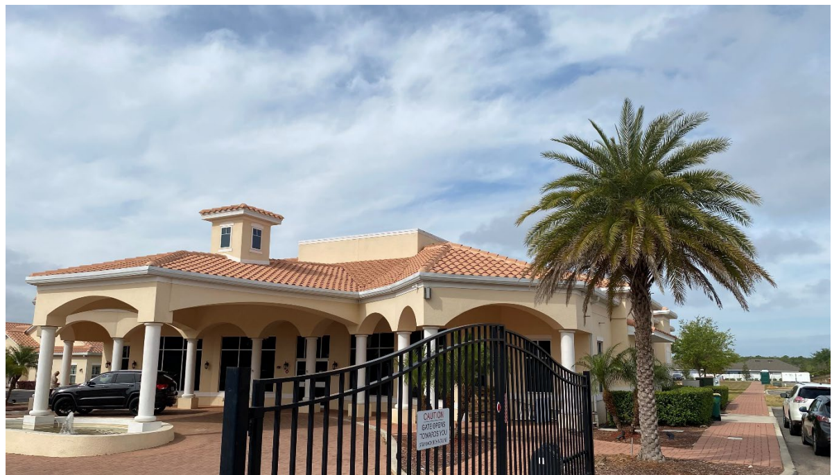
TYPICAL EXTERIOR VIEW OF CLUBHOUSE
