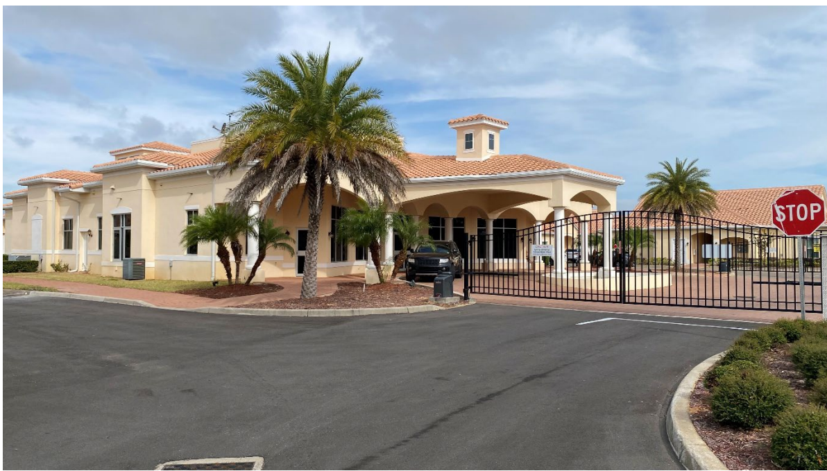
TYPICAL EXTERIOR VIEW OF CLUBHOUSE
